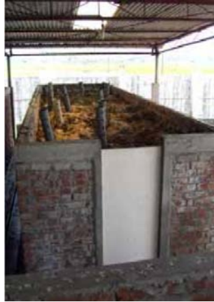
Figure 13. The box composting decentralized composting solution implemented in Dhaka (Source: Waste Concern)
