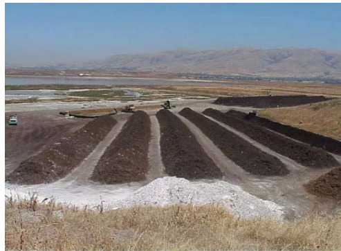
Figure 5. Basic windrow composting
