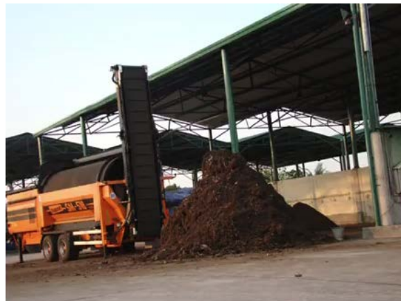
Figure 14. The centralized composting solution implemented in Dhaka (Source: Waste Concern)
