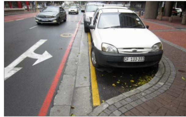
② Parking Lay-by (2.3 m width)
